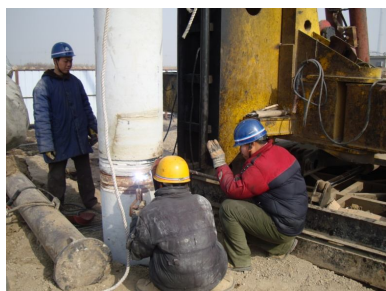
图 9 焊接接桩现场 Fig.9 Welding piles in the field
